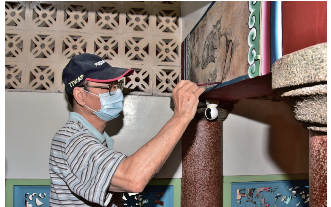
▲Figure 2-17 Painting and restoration of Wanan Temple in Shigang
