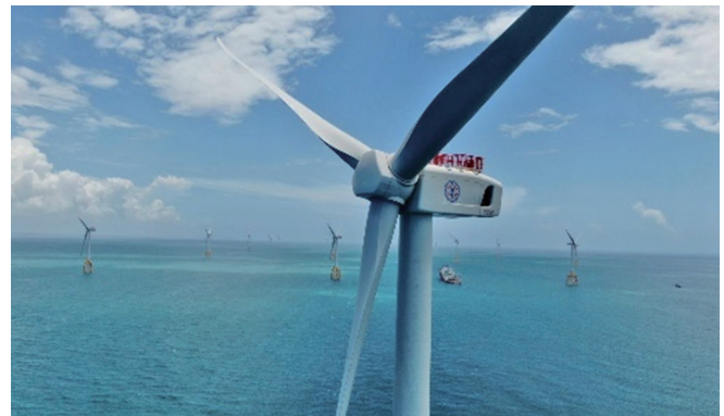
▲ Figure 2-9 Taipower's offshore wind farm in Changhua formally began operation at the end of 2021
