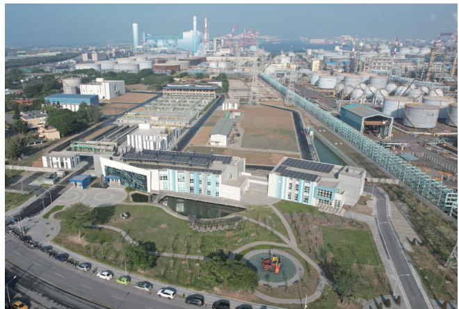
▲Figure 2-8 Kaohsiung Linhai Wastewater Treatment Plant
